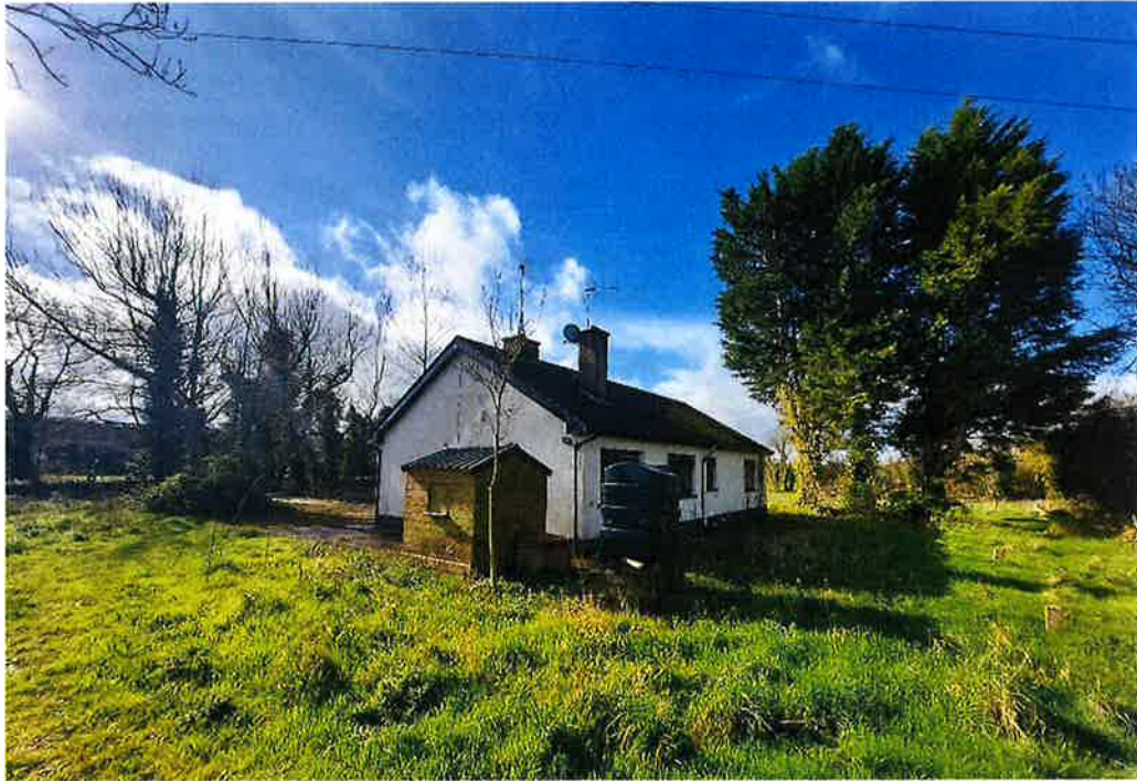
Figure 2.0 Rear view of the existing dwelling (photo taken 27/03/2024)
