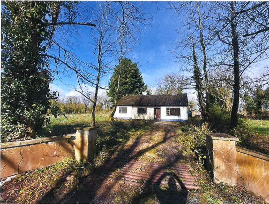
Figure 1.0 Front view of the existing dwelling (photo taken 27/03/2024)
